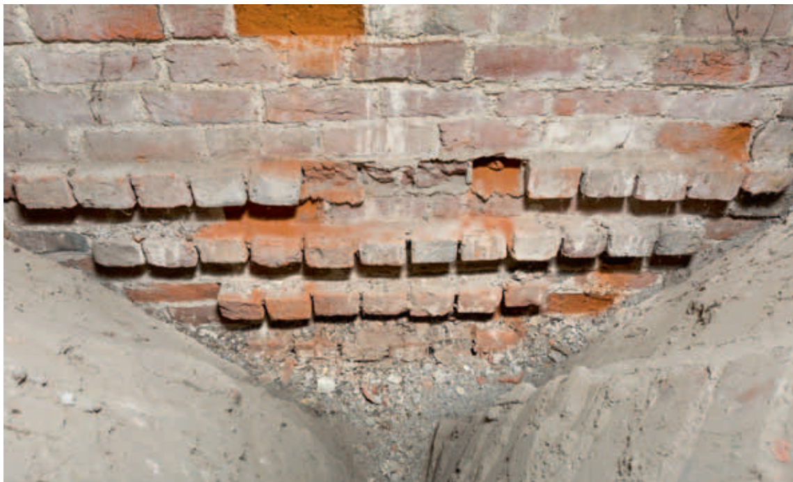
Fig. 23. Hvælvfortanding øverst i korets sydvæg, set fra loftet mellem de to hvælv (s. 1376). Foto Arnold Mikkelsen 2015. – Vault toothing at top of south wall of chancel, seen from the ceiling between the two vaults.
