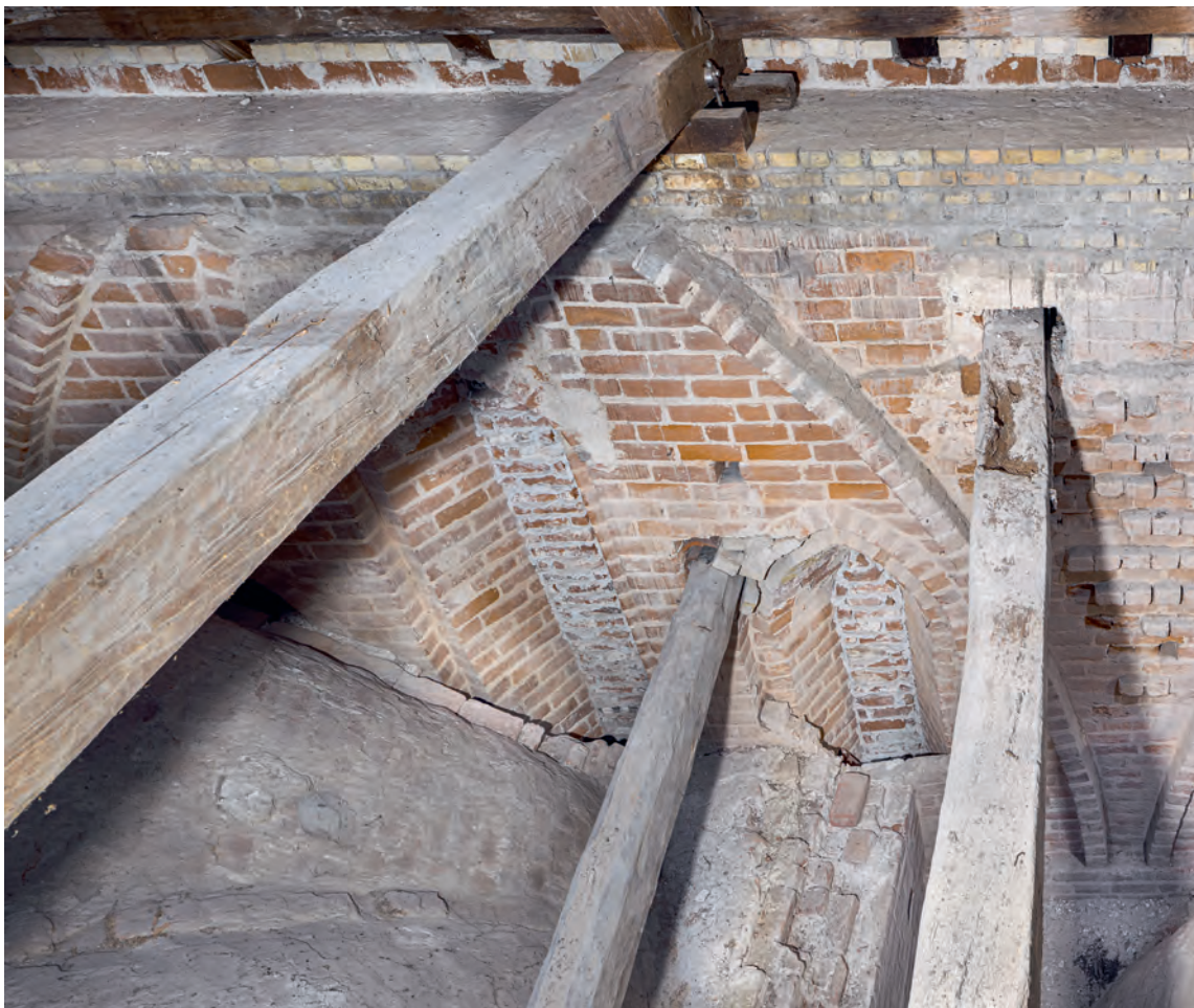
Fig. 49. Søndre højkirkemurs 3. vinduesfag og hvælvfortanding mellem 3. og 4. fag set mod syd (s. 3357). Foto Arnold Mikkelsen 2021. – The third window bay of the southern high church wall and vault tothing between the third and fourth bay, looking south.
