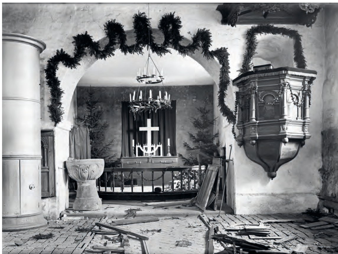
Fig. 44. Indre set imod øst under restaureringen 1912. Foto Hugo Matthiessen. – Interior looking east during restoration of 1912.
